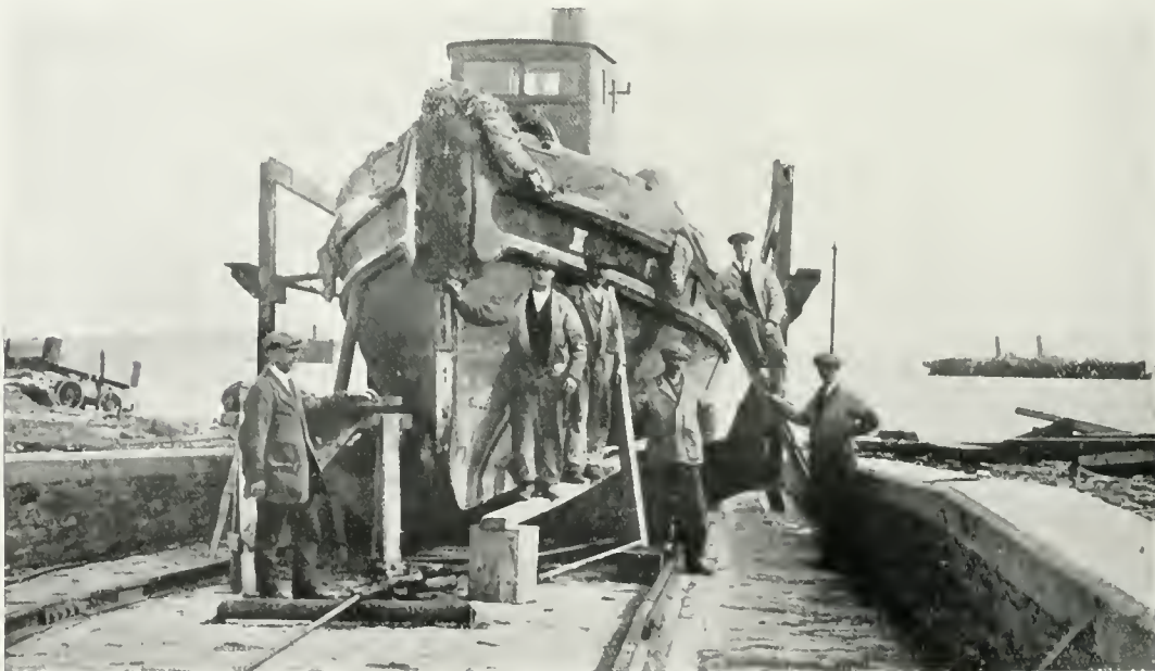
REPAIRING A STEAM PINNACE ON THE SLIPWAY AT LYNESS.
